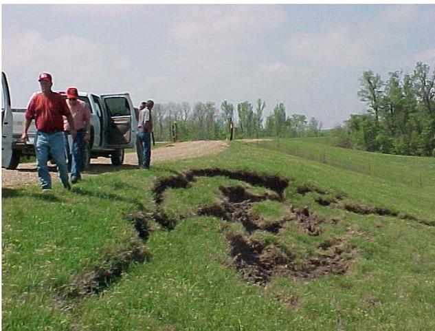
Figure 1: Developing Slide in the Mississippi River levee system (Credit: MS Levee Board)
